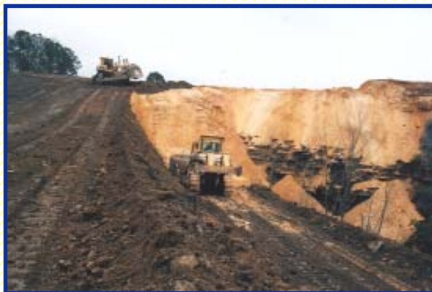
An AML contractor is using bulldozers in backfilling a dangerous highwall in Cullman County.
