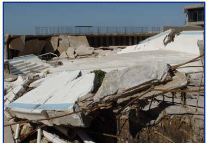
The swimming pool at Gulf State Park Lodge in Gulf Shores was destroyed by Hurricane Ivan. (Photo courtesy of Roger Reetz.)
